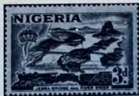
Jebba Bridge and River Niger
